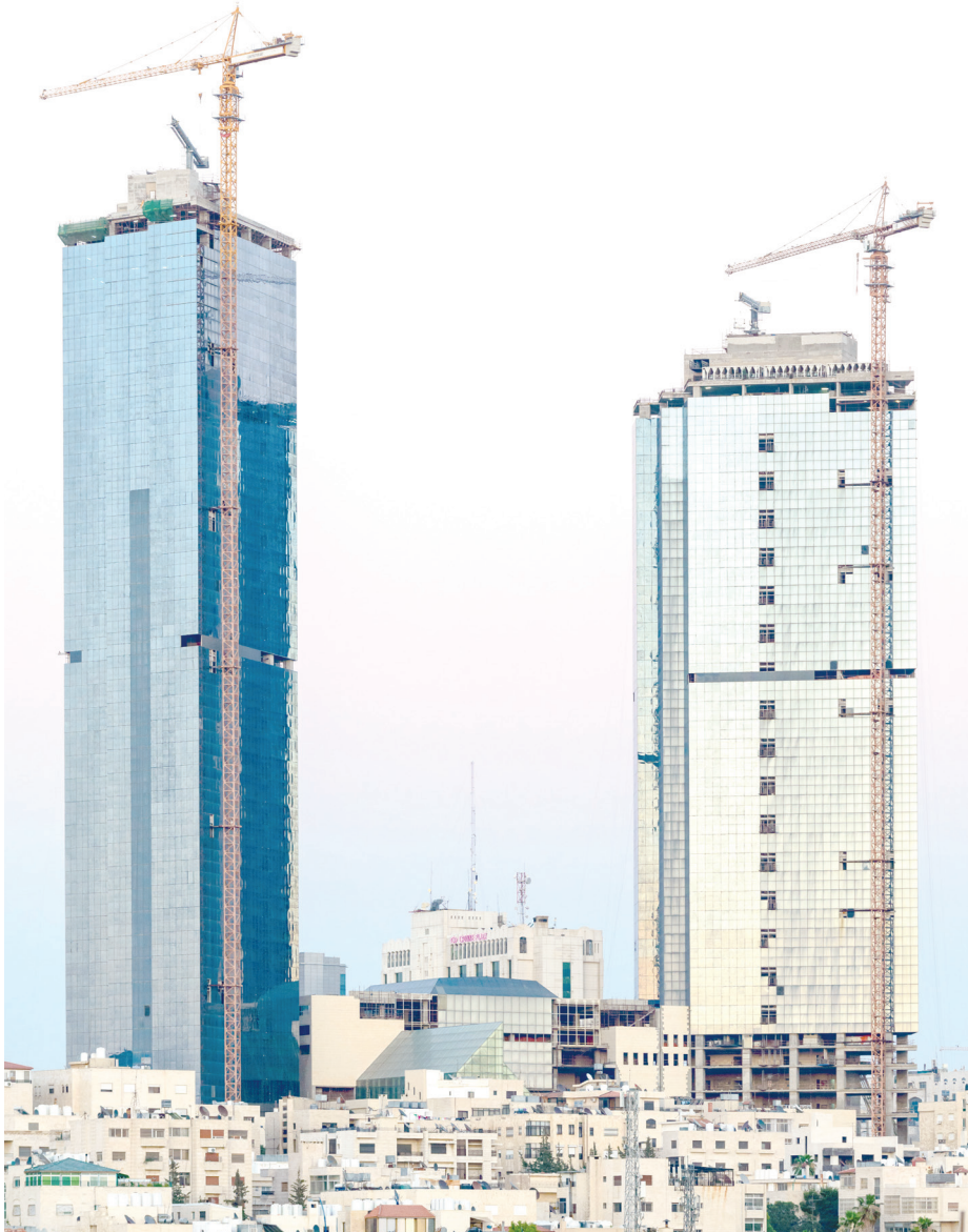
Cranes stand outside the Jordan Gate Towers in Amman. (Photo: Flickr)
